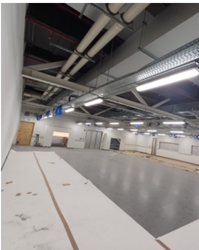
Completed the installation of the rubber floor in CBRA and OSR rooms. This is where our security staff will check the bags.
