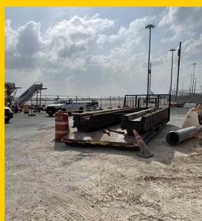
End of October, the works on the sheet pile wall will start. This part of the construction is an important and complicated activity. The sheet pile will be placed on top of 6 meters deep holes that are drilled into the ground. After placing the sheet pile in the holes it will be filled with concrete. This way, an underground wall will be built, supporting both the existing and new building. The sheet piles have already arrived on site, and installation will begin soon.
